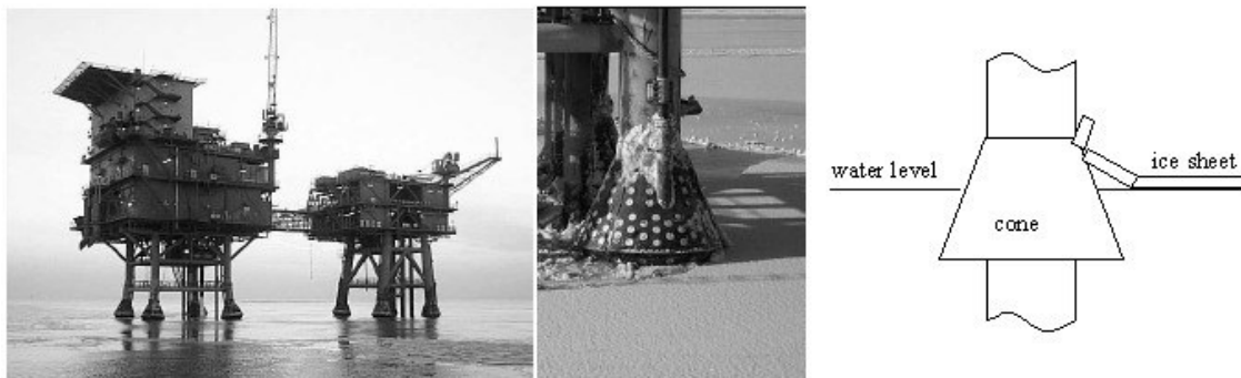
Figure 3: Conical structures attached to oil platform
